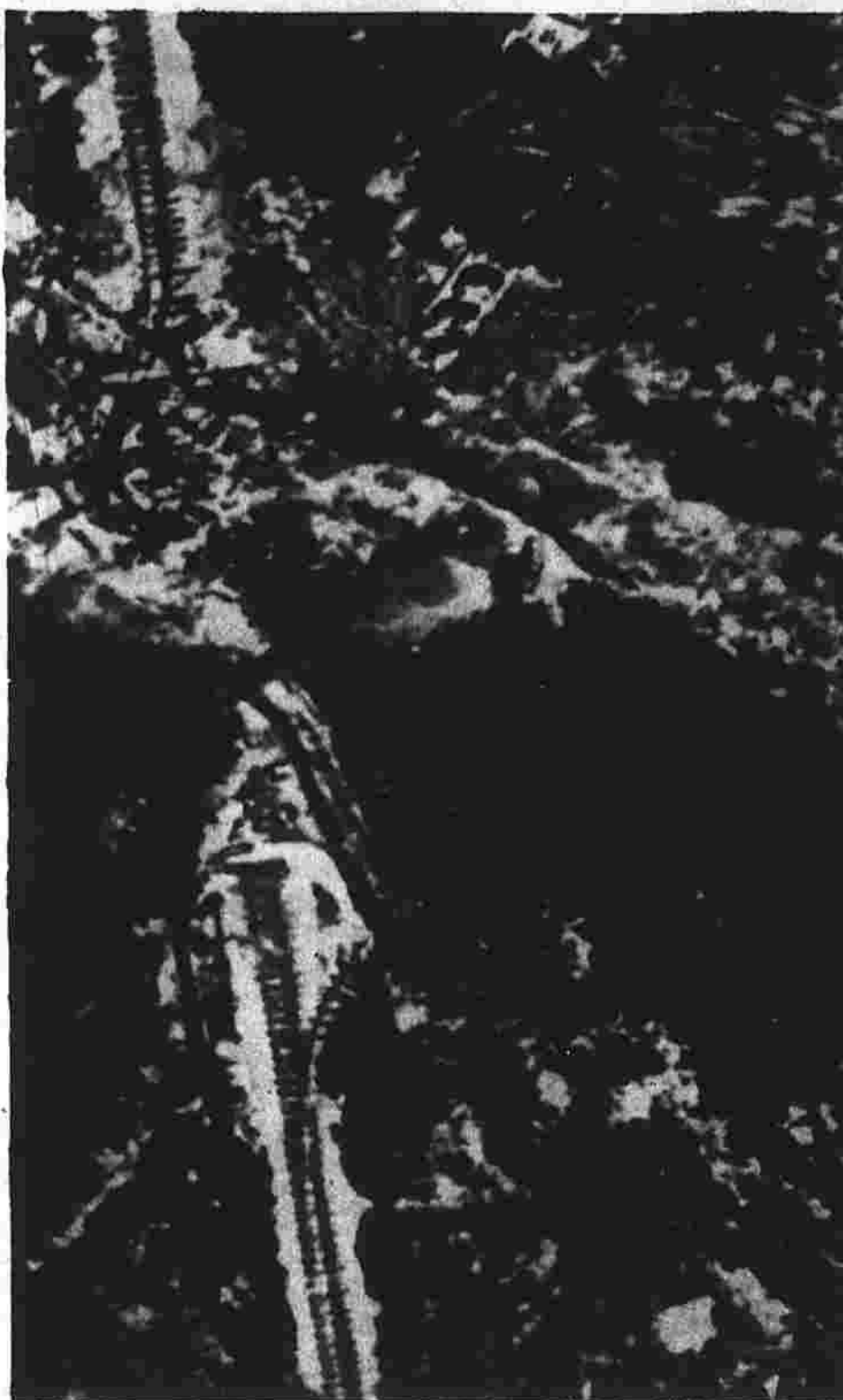
Bridge Out This United States Air Force aerial photo, released Wednesday in Saigon, shows the damaged 96-foot long Vu Chu railroad bridge hit by guided bombs June 22. The bridge, located 38 miles from Hanoi, crossed the Sui Ngang River in North Vietnam. (AP photo)
